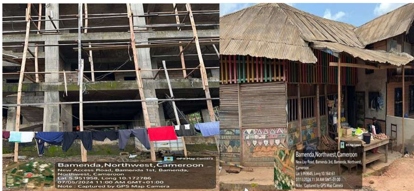
Figure 9: Example of semi-permanent informal housing in Bamenda
