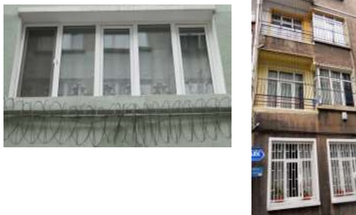
Figure 4. Second or third floor window bars in Cihangir
